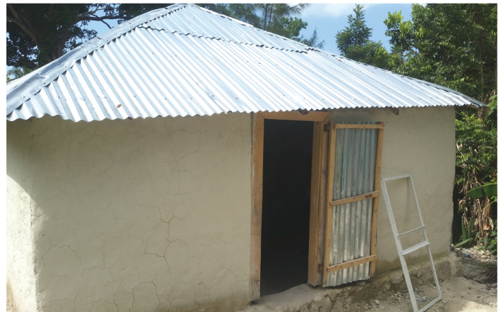
Construction of the new school in St. Martin de Tours.
